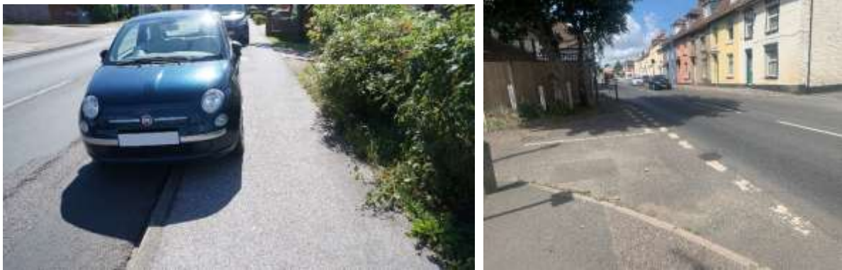
Figure 7-2: Example of footway parking reducing the footway width (Left – Bysing Wood Road) and wide junction radii prioritise turning vehicles and elongate pedestrian crossing (Right – London Road (A2))
